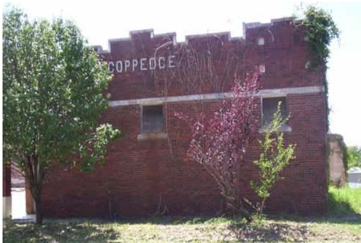
Removal of vines and shrubbery overgrowth reveals lettering that remains intact.
